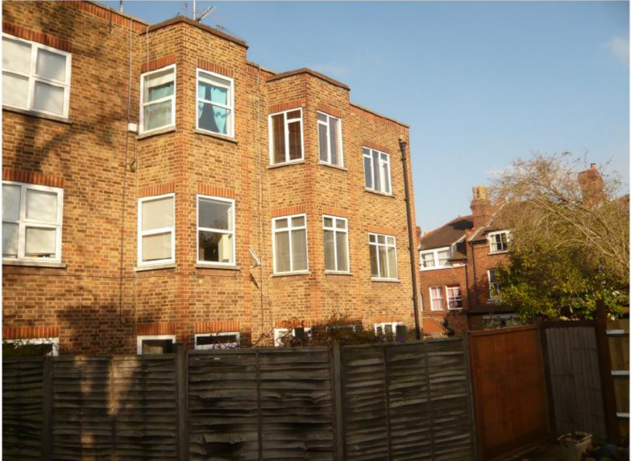
Rear elevation of building
